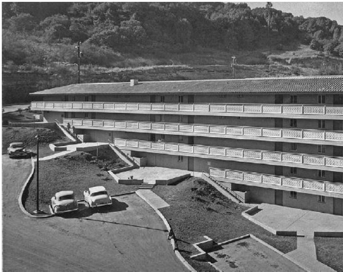
Figure 19. A 1961 image shows evidence of precast concrete curbs rather than the specified redwood headers. Source: Ruark, 2017.
