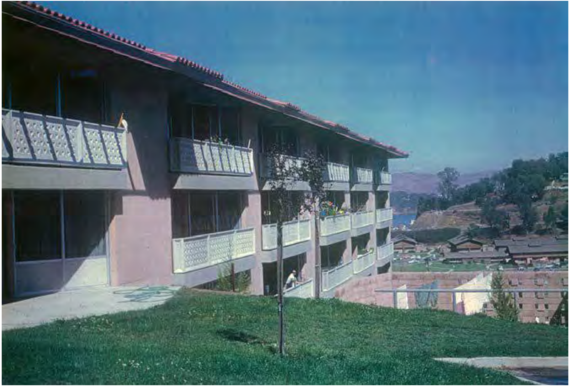
Figure 27. The historic condition of the façade at the rear of the high-rise buildings in 1961, illustrating the precast balcony guardrails with the exposed rafters overhead and the warm clay/pink color of the concrete façade. Source: Ruark, 2017.
